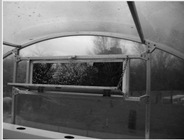
Premier Tunnel House with adjustable vent
